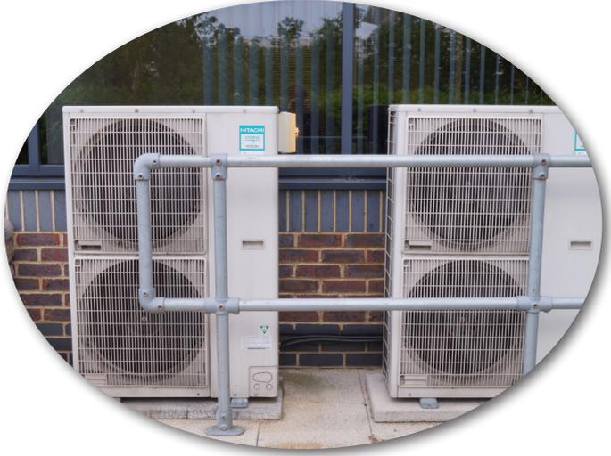
**Air source heat pumps are a very efficient way of providing heat for your hot water or heating system by extracting heat from the air outside and transferring it into a building. They work in a similar way to refrigerators, but in reverse. They are similar in appearance to air-conditioning units.**
